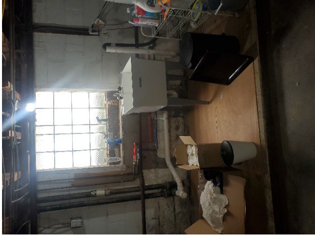
Photo 37: View of the laundry area in the Basement of the Rectory.
