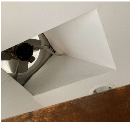
Overcroft ventilation fan detail and context (courtesy of WC Keller)
