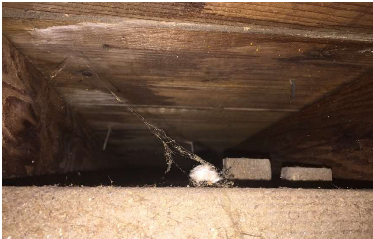
Rectory wall cavity as seen from attic in rectory
