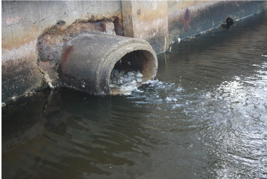
Figure 13 - Outflow into Manchester Waterway
